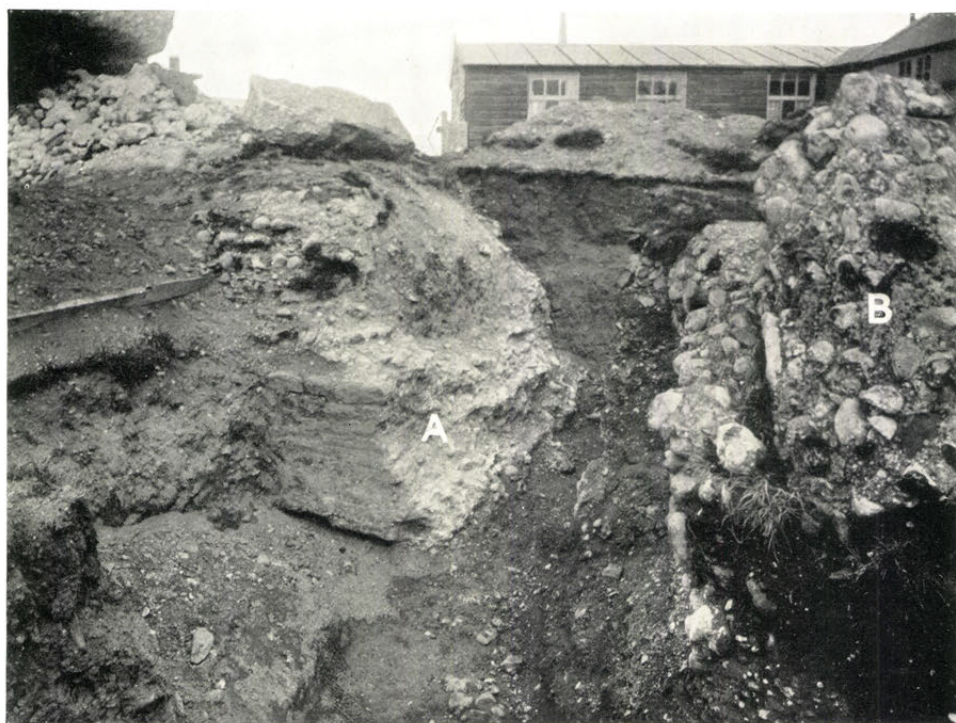
Fig. 2. Site of south postern turret, p. 33 A. broken end of main wall; B. fallen masonry
