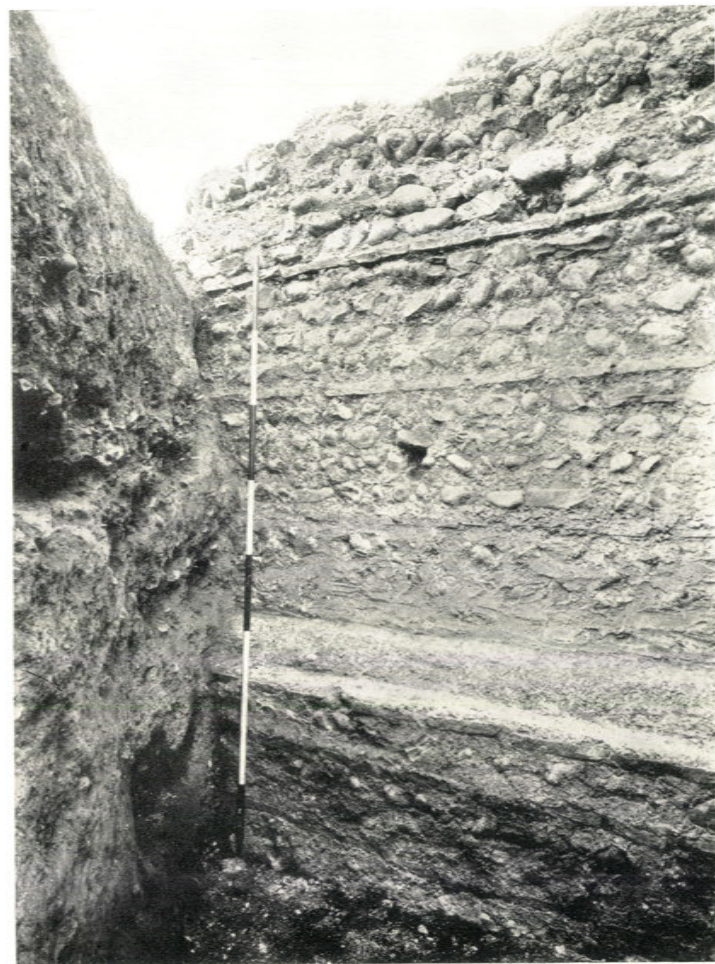
Fig. 2. Face of north wall of fort, p. 20
